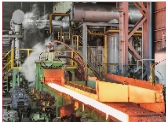
Medium Section Mill modernization
